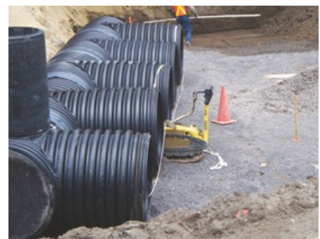
PREPARING THE SOIL FOR HDPE PIPE INSTALLATION
