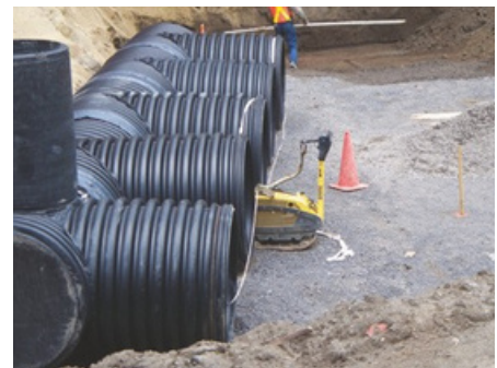
PREPARING THE SOIL FOR HDPE PIPE INSTALLATION
