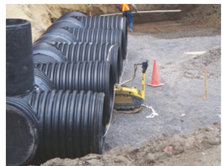
PREPARING THE SOIL FOR HDPE PIPE INSTALLATION
