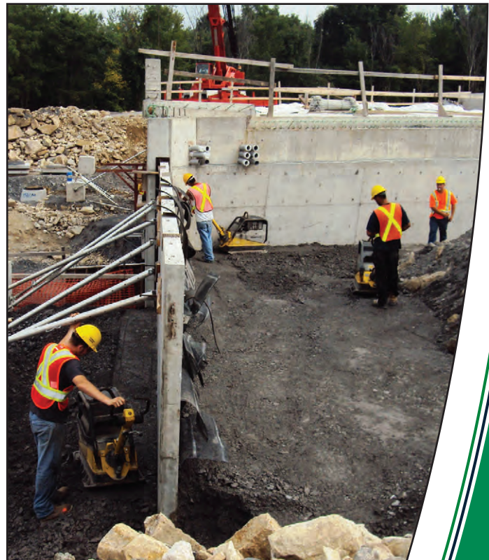
Step 4 - Backfill and compact
