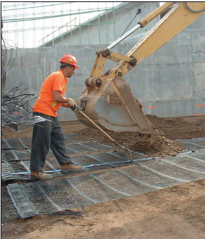
Step 3 - Connect and place geogrid
