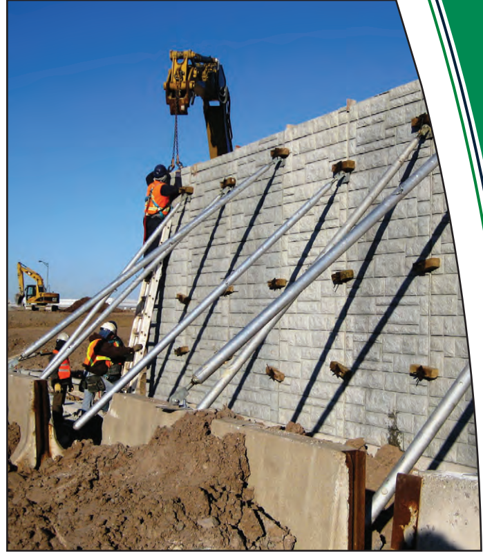
Step 2 - Place and brace panels
