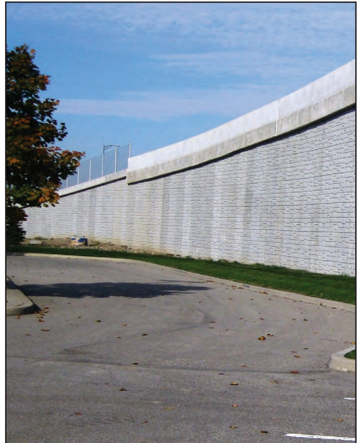
Traffic Barrier & Fence
