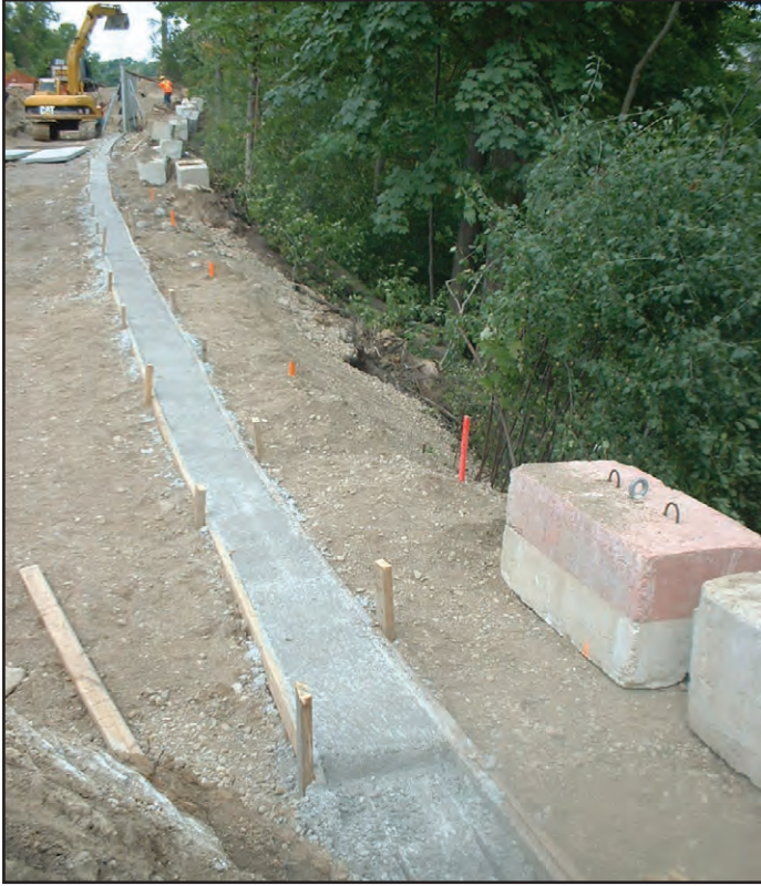
Step 1 - Prepare subgrade and cast footing/leveling pad
