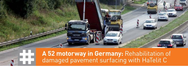
The repair works commissioned by Landesbetrieb Straßenbau NRW – the state enterprise responsible for highway maintenance in the German State of North Rhine-Westphalia – to the damaged pavement surfacing on the section of Germany's A 52 motorway between the Neersen and Mönchengladbach interchanges were carried out in July 2009 using HaTelit C. The first step was to mill off the existing surface course and binder course.
